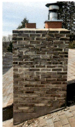
BEFORE: Missing mortar joints, spalled brick facing, cracked mortar wash crown, and gaps in flashing.
